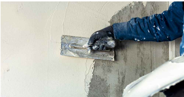
Cement Plastered Walls
