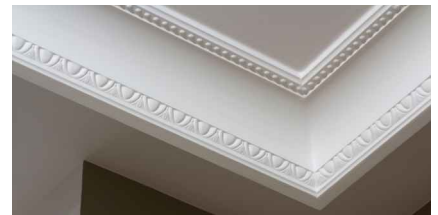
P.O.P-Based Decorative Moldings And Wall Structures
