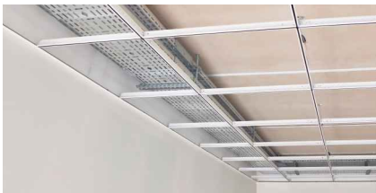
False Ceiling Installations
